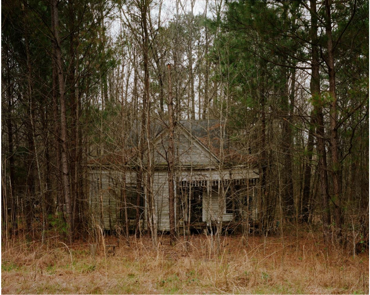
Abandoned House, William Faulkner Memorial Highway, Mississippi, 2020
